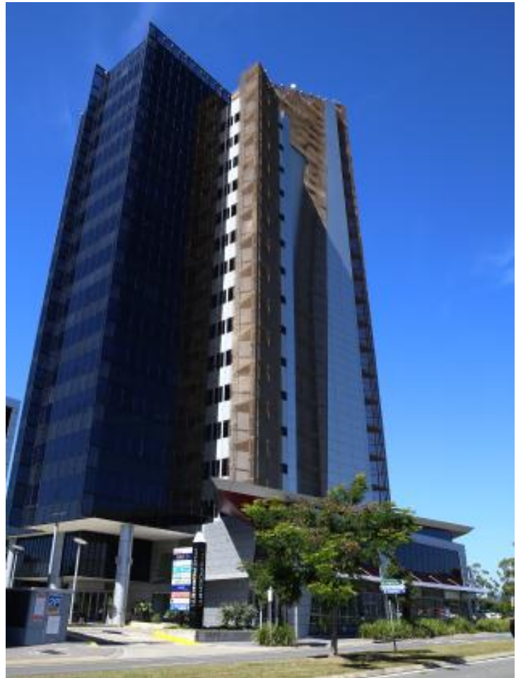
📷 The Rocket building at Robina where Members Alliance have been failing to pay rent. Photo: David Clark
